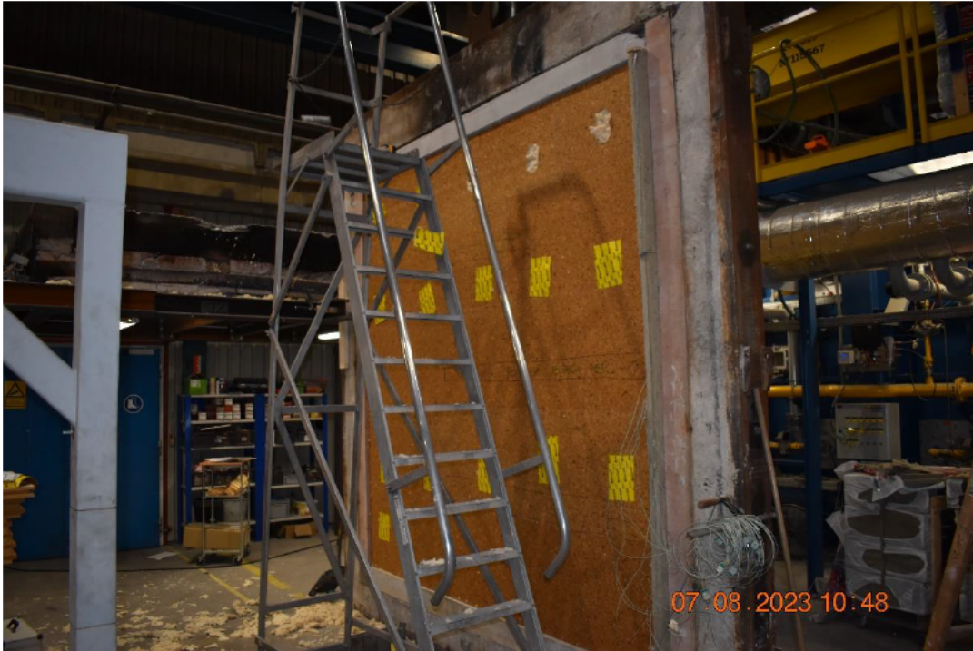
Photo No. 7 Inner layer seen from unexposed side
