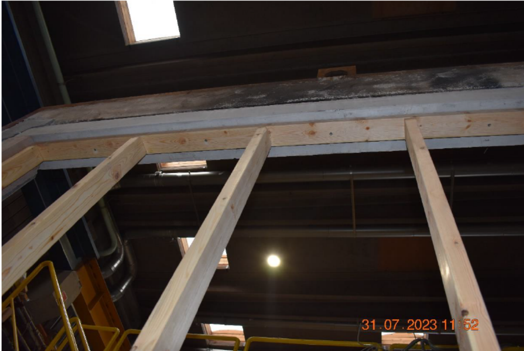
Photo No. 1 Wooden frame in test frame
