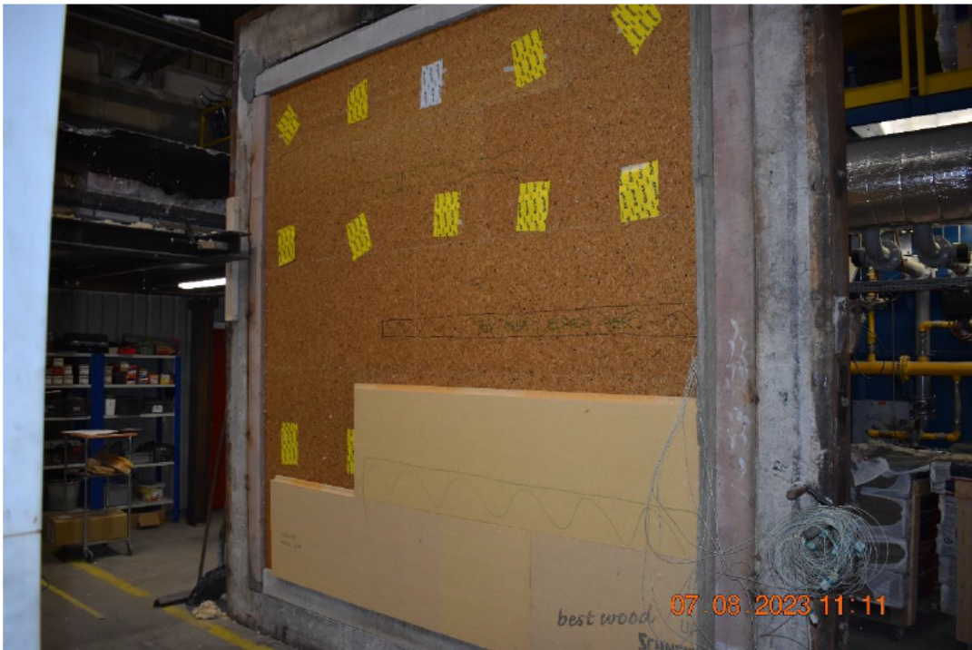
Photo No. 8 Outer layer during mounting seen from unexposed side
