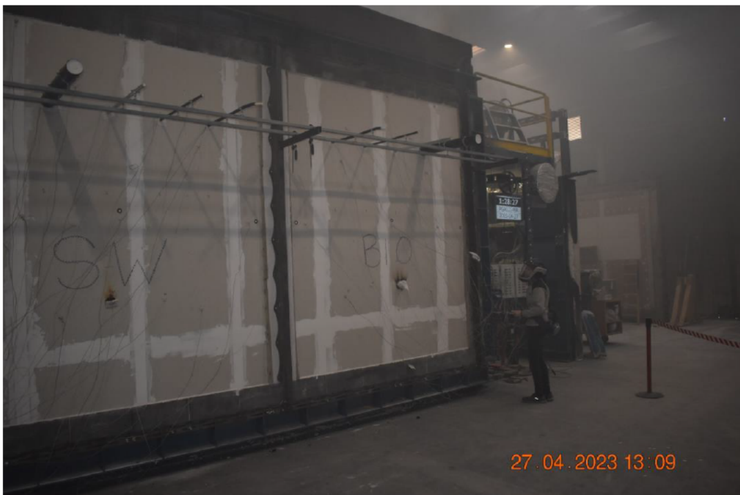
Photo No. 18 Test specimen seen from unexposed side after 88 minutes of testing
