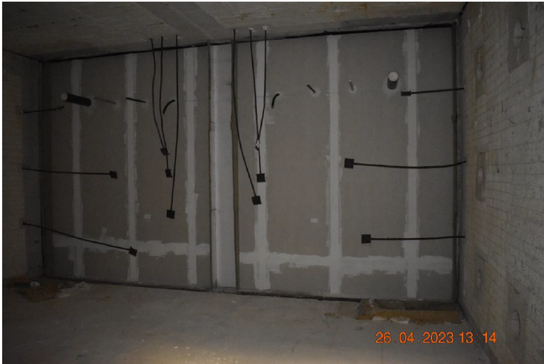
Photo No. 7 Test specimen seen from exposed side before test start
