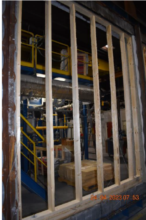
Photo No. 1 Supporting construction wooden frame during mounting
