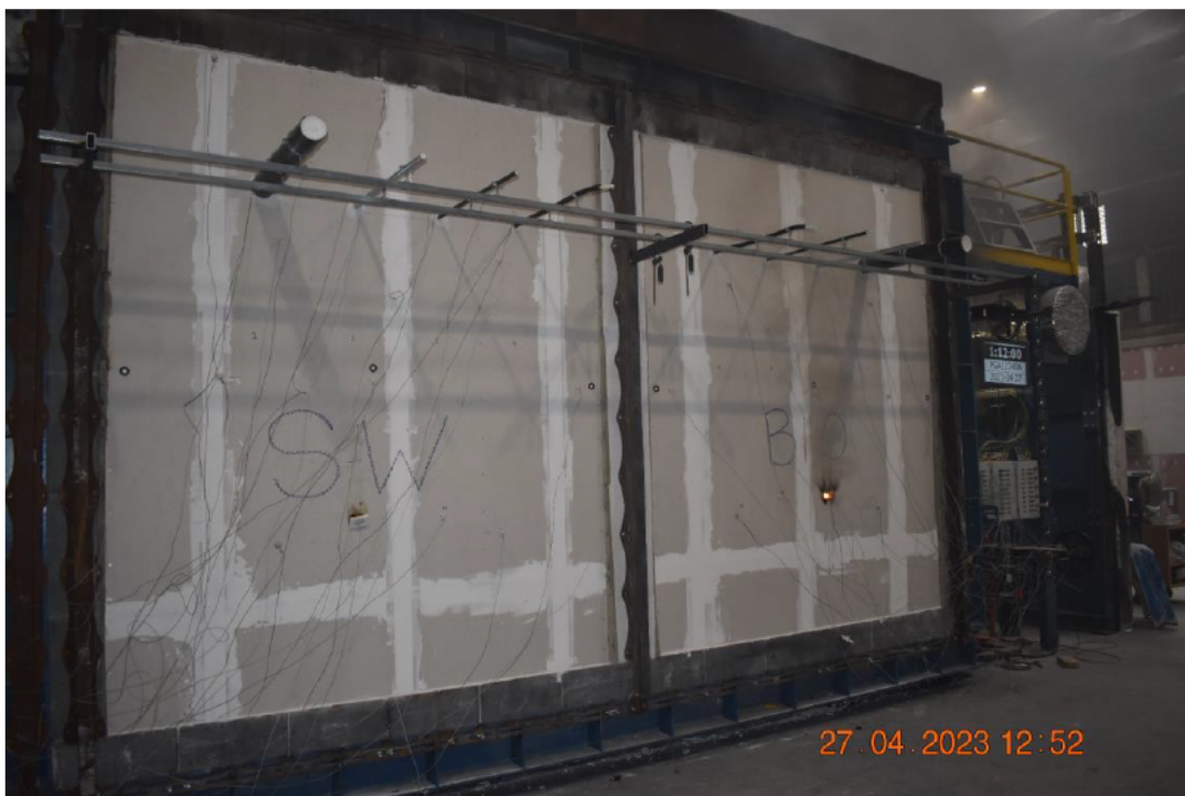
Photo No. 16 Test specimen seen from unexposed side after 72 minutes of testing
