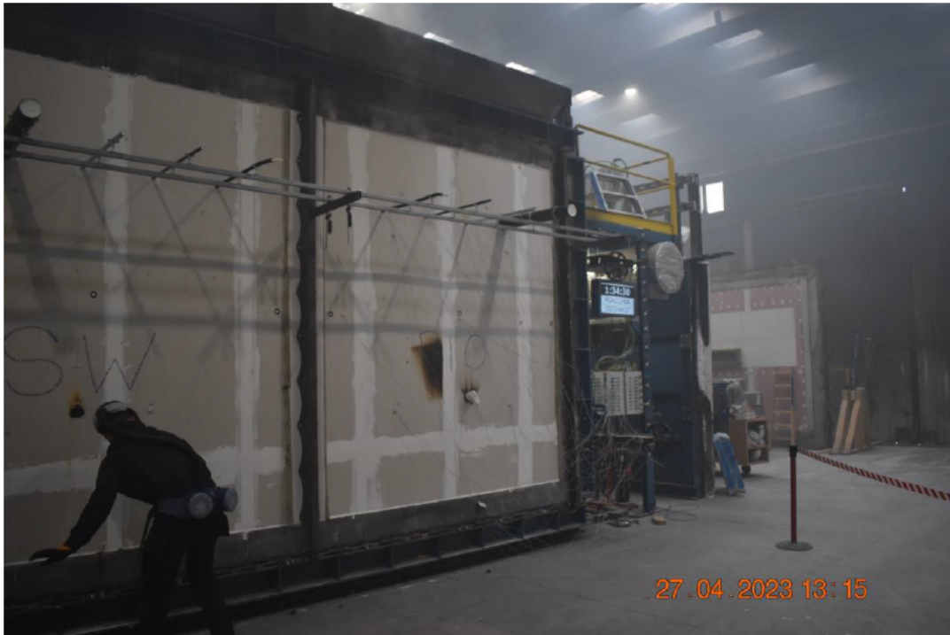
Photo No. 19 Test specimen seen from unexposed side after the test
