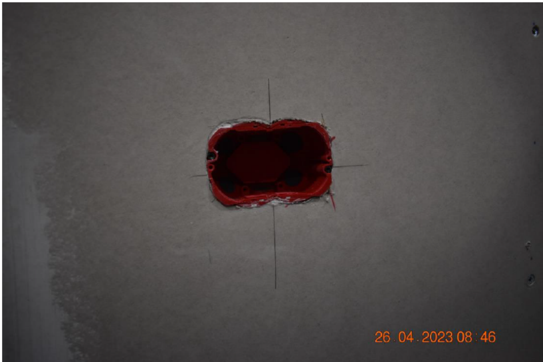
Photo No. 8 Installation box during mounting
