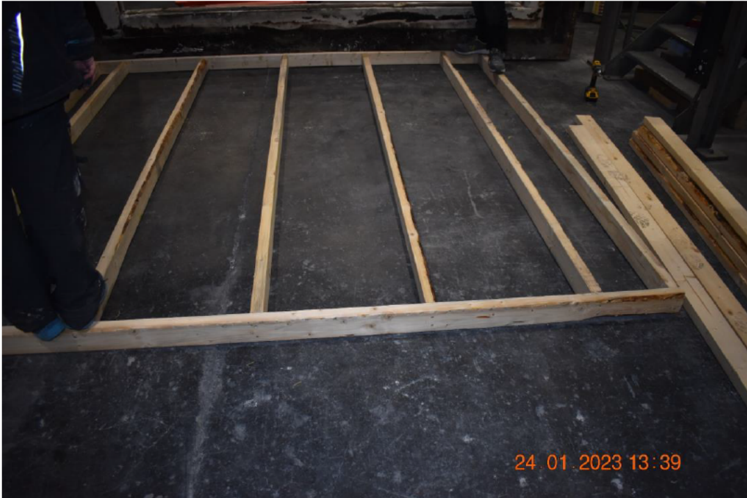
Photo No. 1 Wooden structure during assembly
