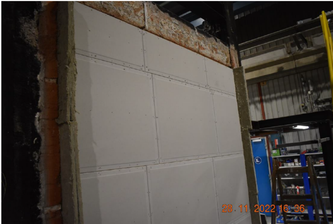
Photo No. 7 Mounting of fiber gypsum boards
