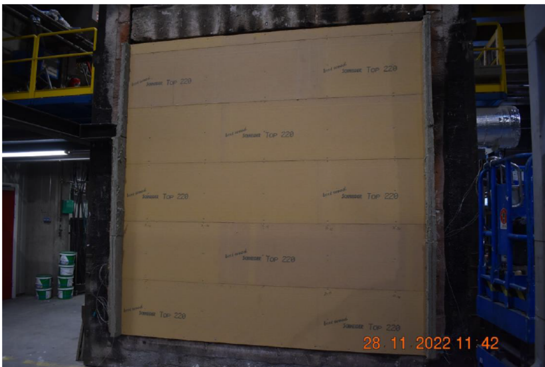
Photo No. 4 Wood fiber board mounted on unexposed side
