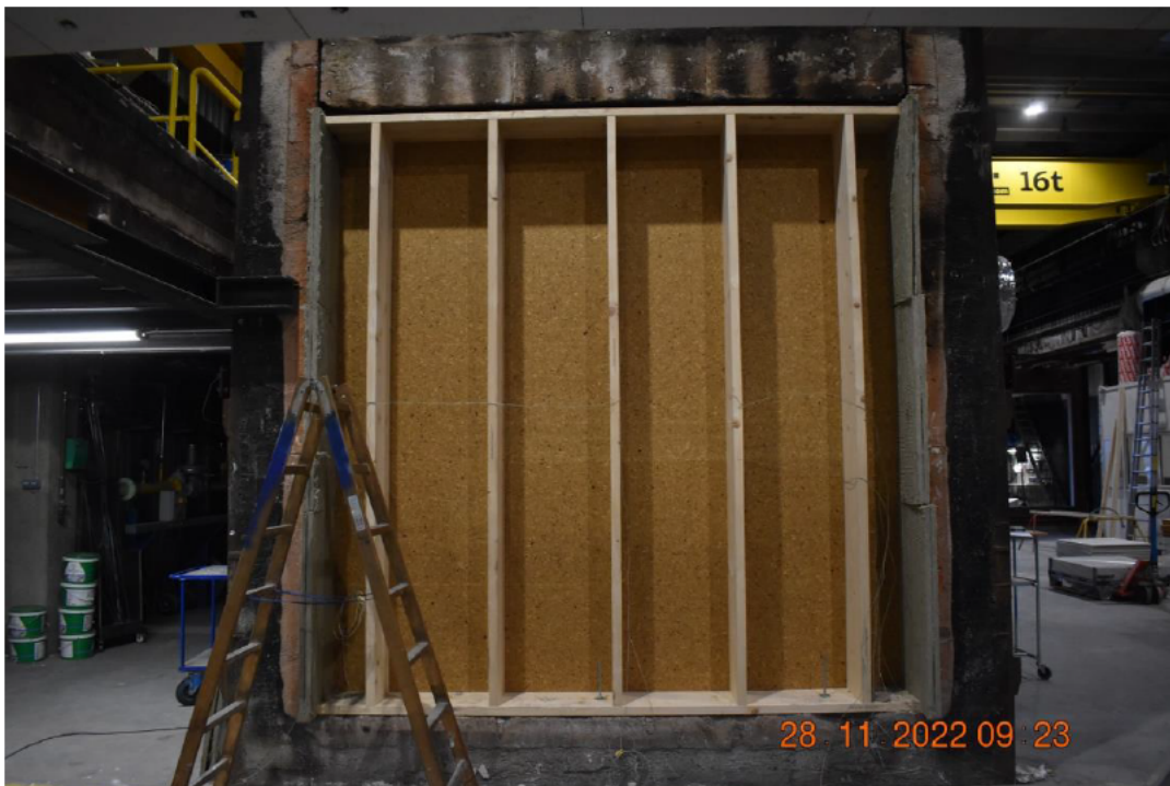
Photo No. 2 Chipboard mounted on one side
