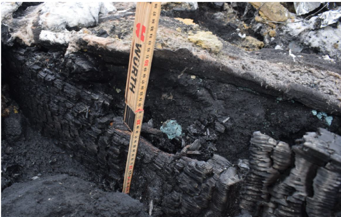
Photo No. 20 Wooden stud measurement after the test
