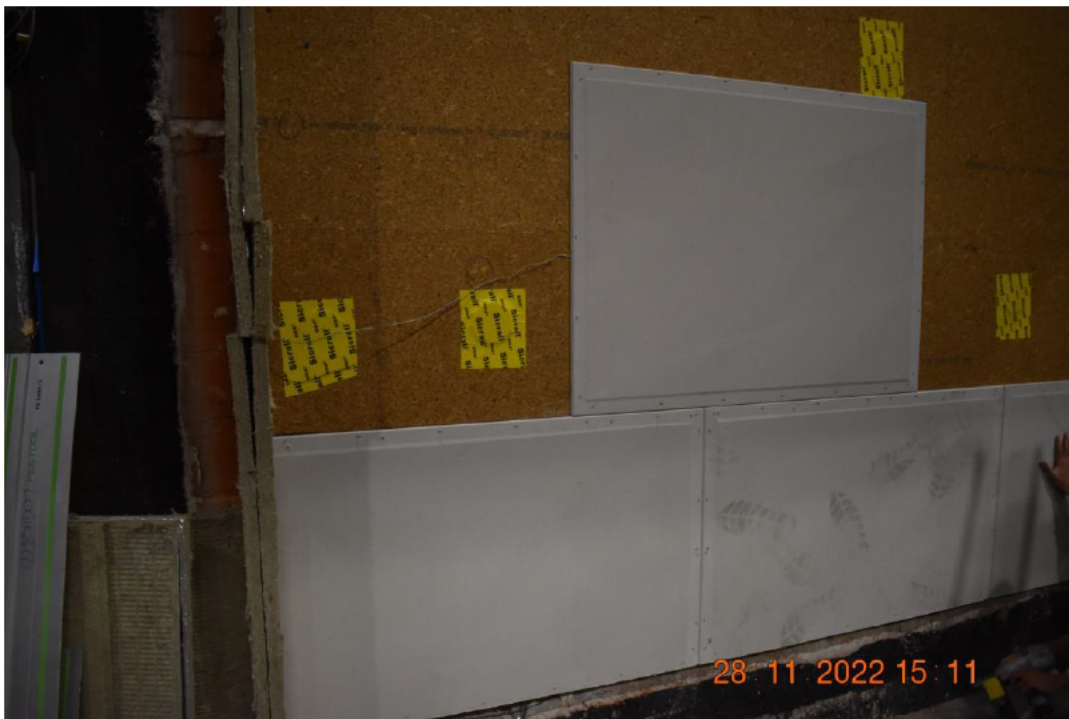
Photo No. 6 Mounting of fiber gypsum boards
