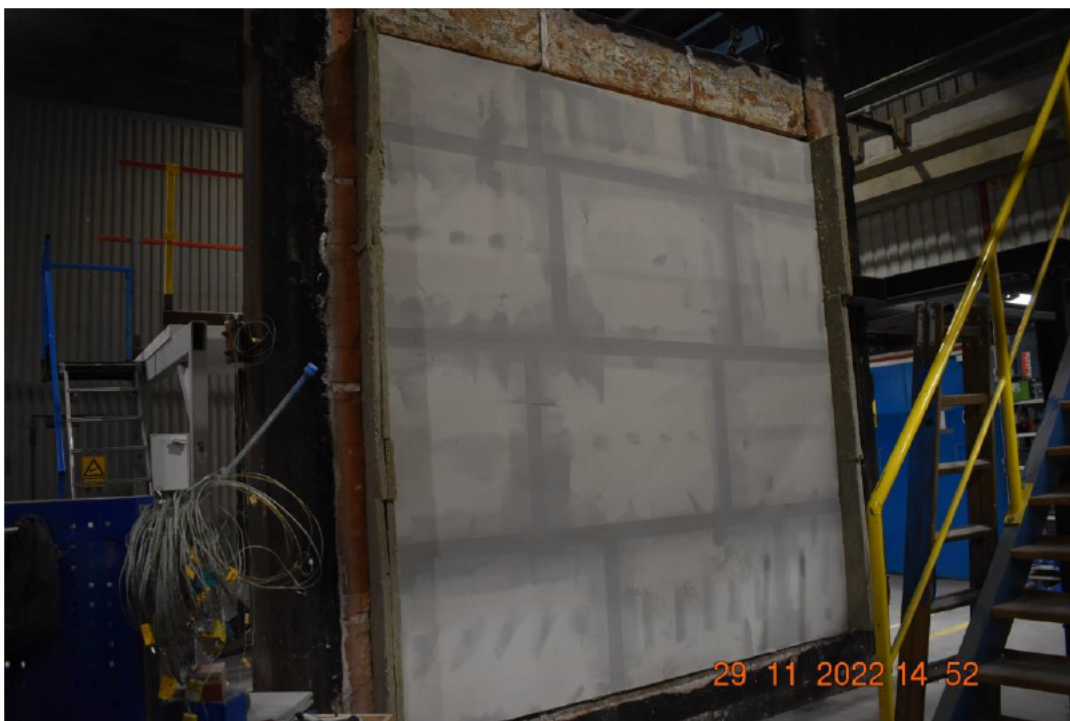
Photo No. 8 Filler is applied on the fiber gypsum boards
