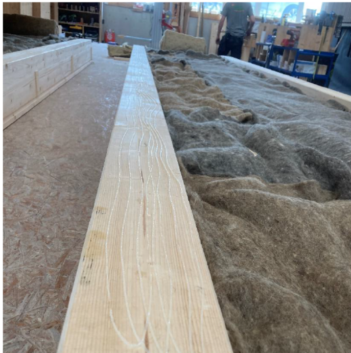
Photo No. 4 Glue applied on timber beam before mounting the CLT-element
