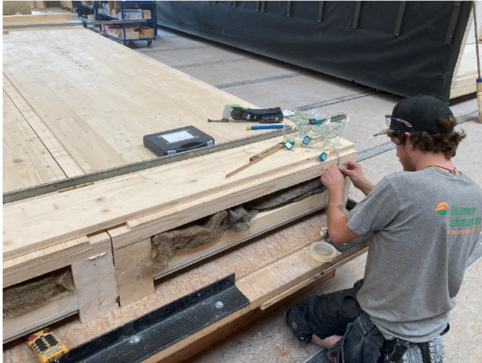
Photo No. 7 Both elements glued and fitted together
