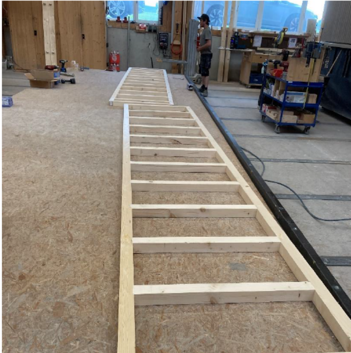
Photo No. 1 Timber battens before mounted between timber beams
