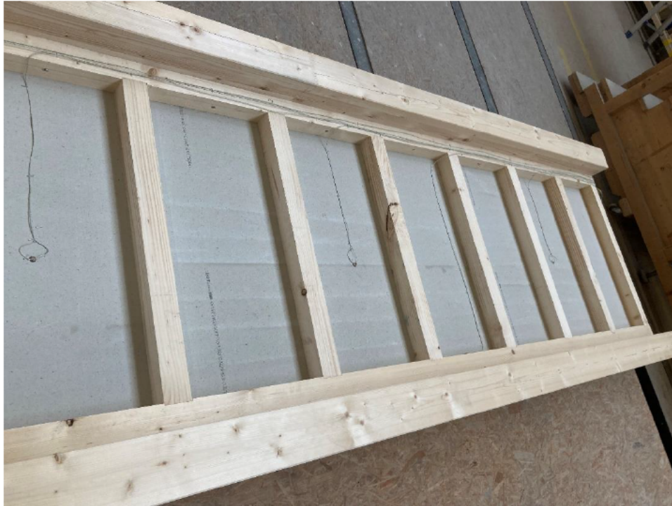
Photo No. 3 Timber battens and beams mounted.
