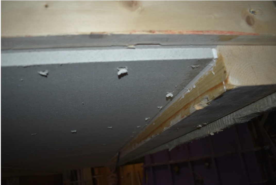
Photo No. 19 Seal after removal of excessive sealant
