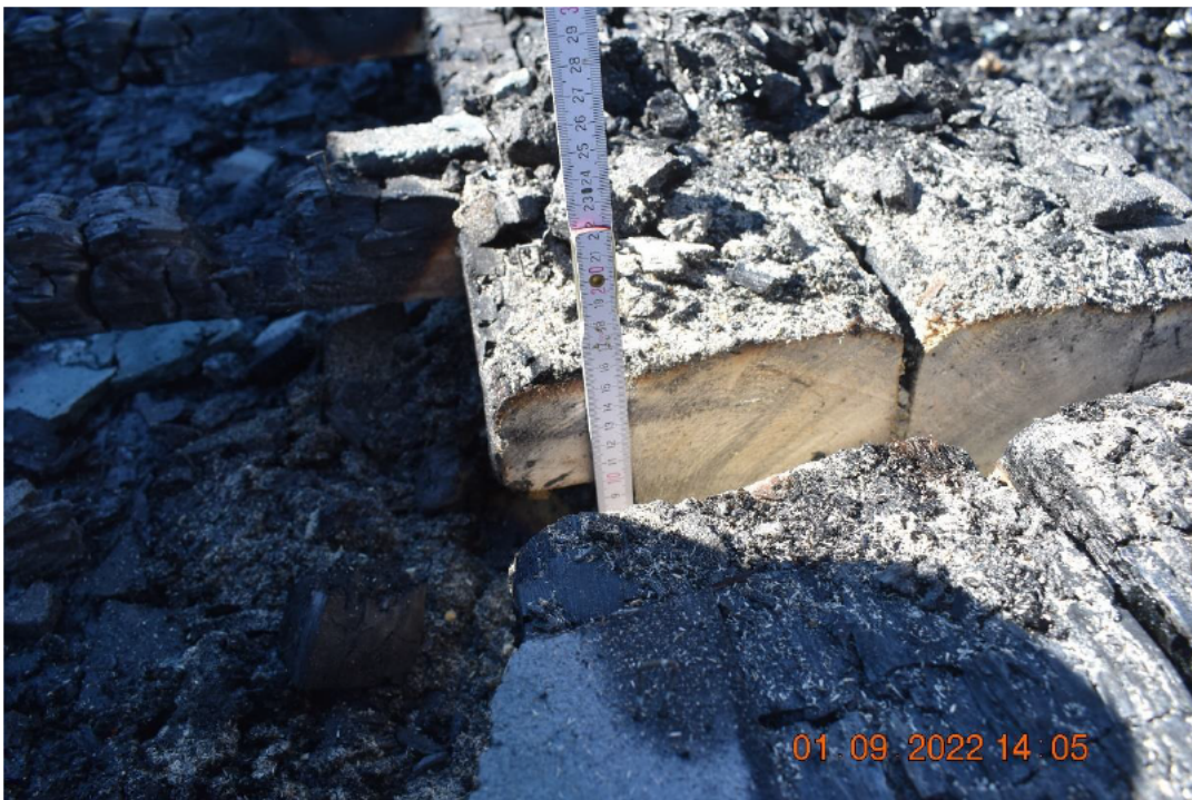
Photo No. 36 Charring of centre timber beams after test
