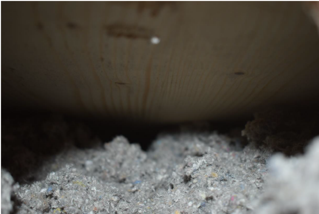
Photo No. 16 Close-up on the insulation inside the element
