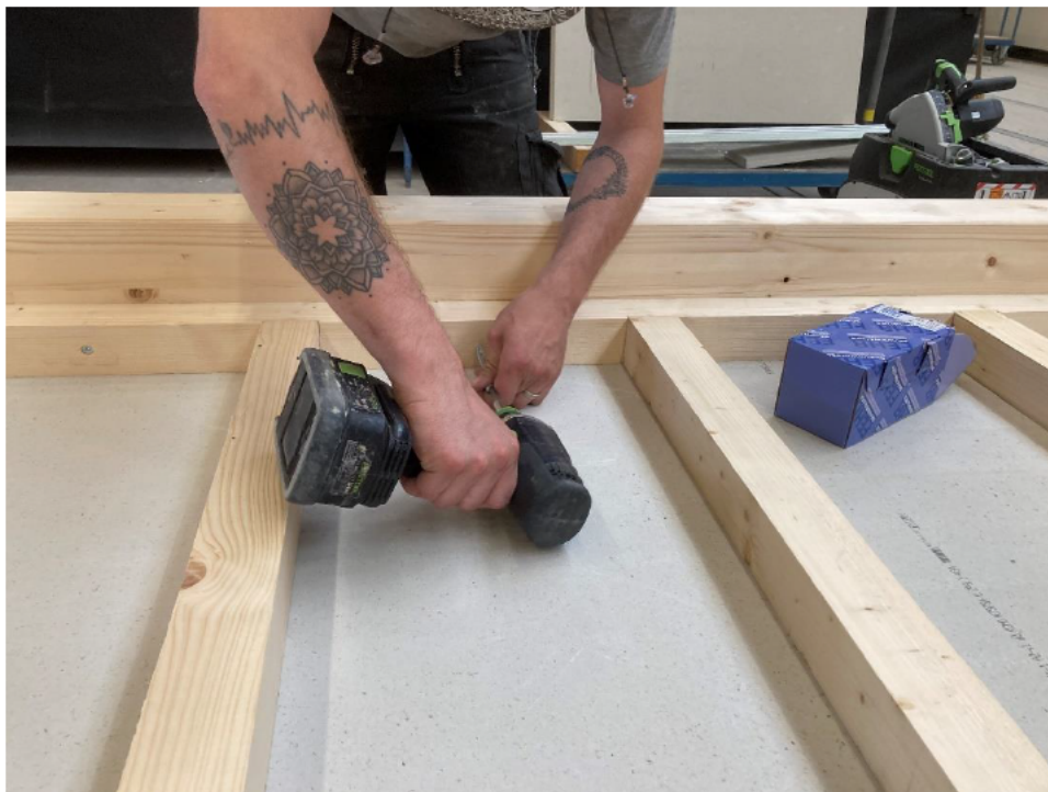
Photo No. 2 Timber battens being fixed to the timber beams
